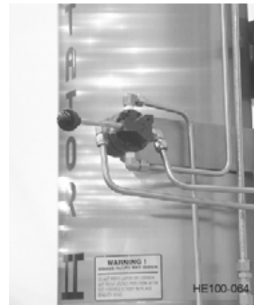
Figure 15 - Direction Valve
