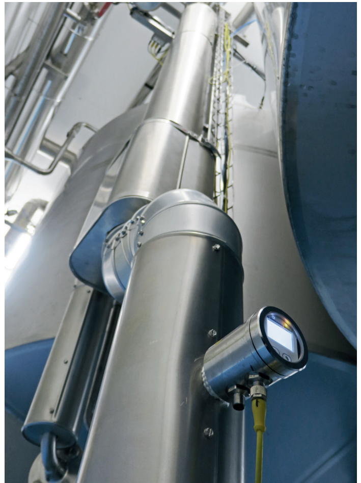
The activation of the cleaning agent concentration in a separate circulation is monitored with an ILM-4.
