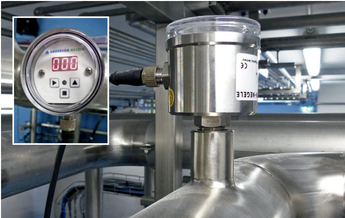
The compact flow monitors FTS monitor the return flow of the media.
