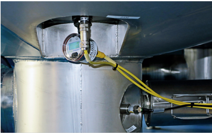
Volume, temperature and level measurement of tank contents with L3, TSM and LS
