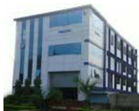
Tecnik Fluid Controls Pvt. Ltd. Mumbai, India
